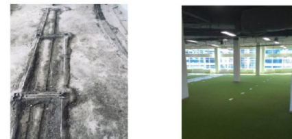
6. Kazakhstan factory flooring
